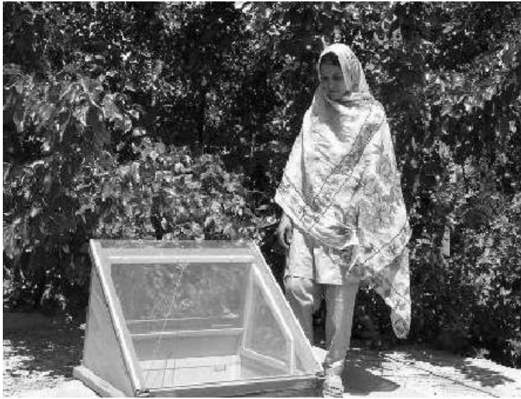
Figure 14.7 BACIP Roof Hatch Window to Cover the Roof Opening
