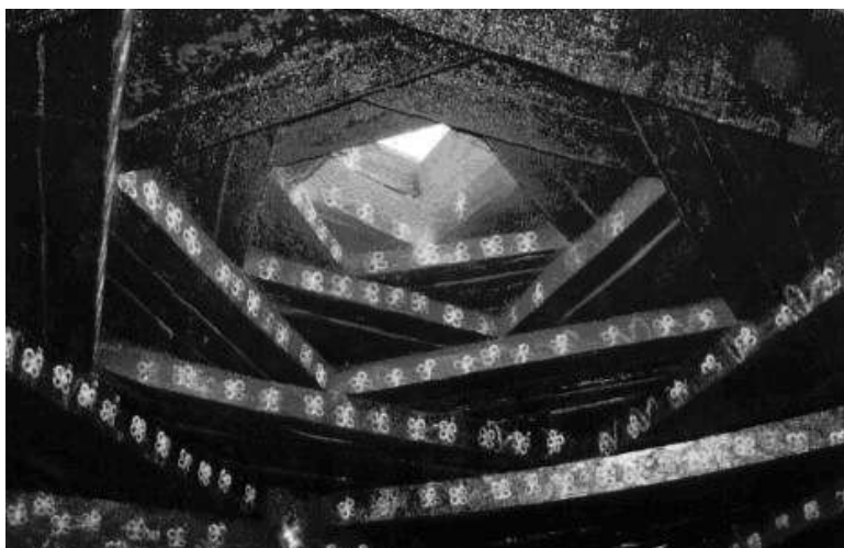
Figure 14.5 Roof Opening in the Traditional House (inside)
